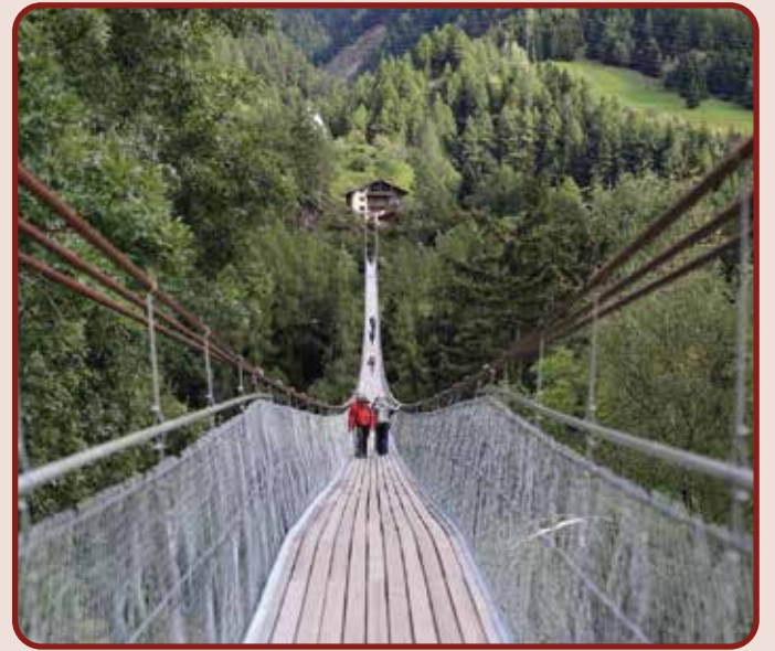
Goms Bridge, Goms, Kanton Wallis
